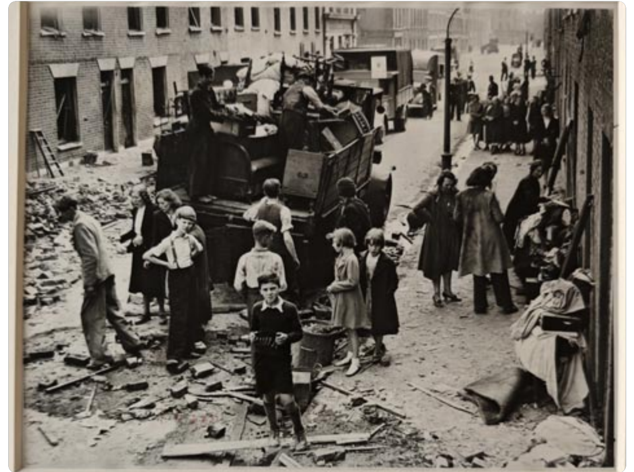
Keystone Agency Last Night's Raid Damage, London, 28 July 1941
